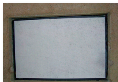
A deck with added firewall
